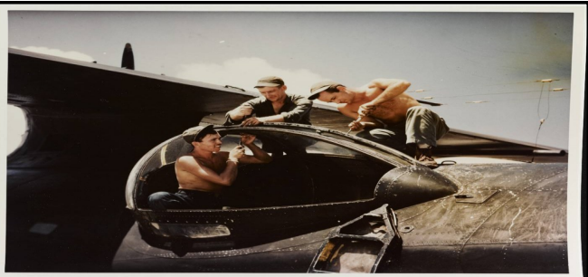
(Left) A Consolidated PBV-5A Catalina Patrol Aircraft receives repairs to a gun blister at a Pacific Navy repair base, April 1945.
